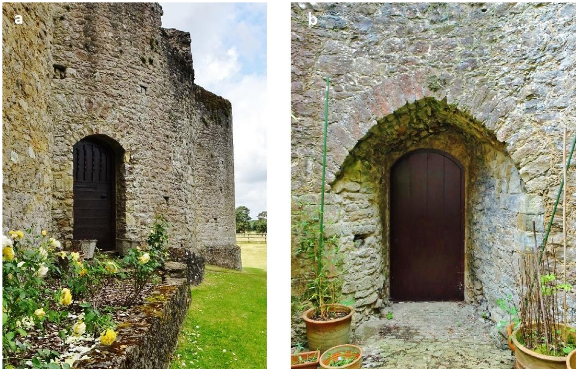
Fig. 82: Leybourne Castle gatehouse east tower, altered northeast loop G9, now a doorway: a) external view, from east; b) internal view, from southwest
