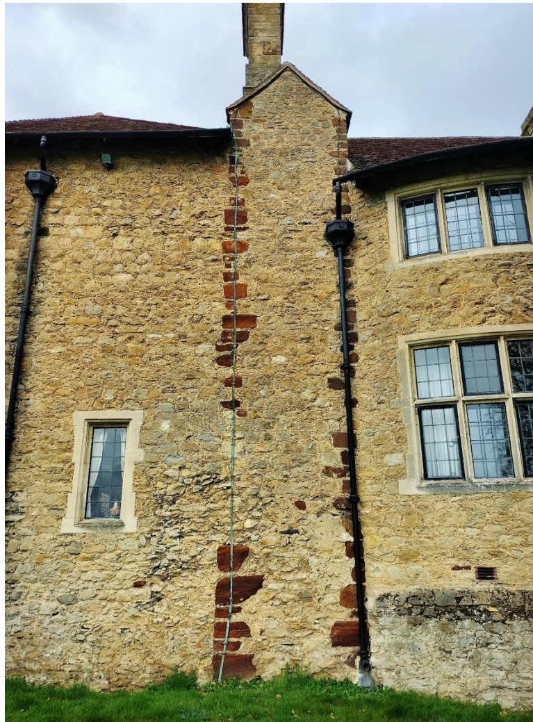
Fig. 101: The present house, exterior of east wall. Left to right: square-headed light, possibly medieval in origin; quoined strip (end of chamber-block north wall?); semicircular bay with basal plinth
