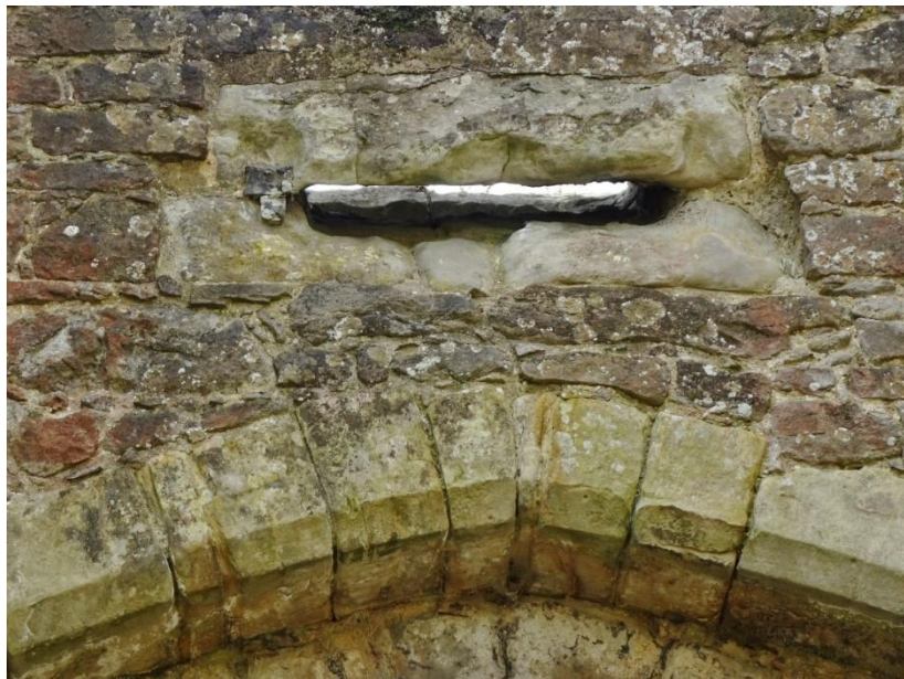
Fig. 59: Leybourne Castle gatehouse: the 'letterbox chute' over the entry, from north
