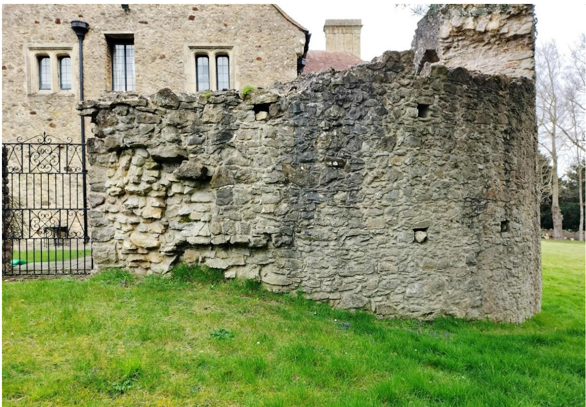
Fig. 90: The Southeast Tower from south, showing scar from attached ?turret (to left)
