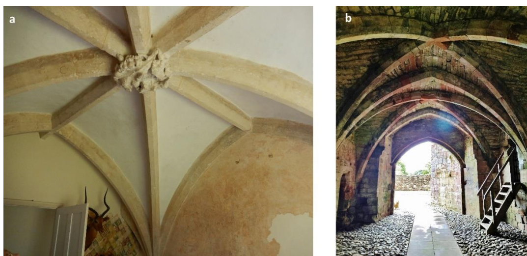
Fig. 123: The quadripartite passage vaults in a) the gatehouse at Bampton Castle, Oxon. (Aymer de Valence, 1315-24), and b) the inner gatehouse at Brougham Castle, Westmorland (possibly Robert de Clifford, c.1300-10)
