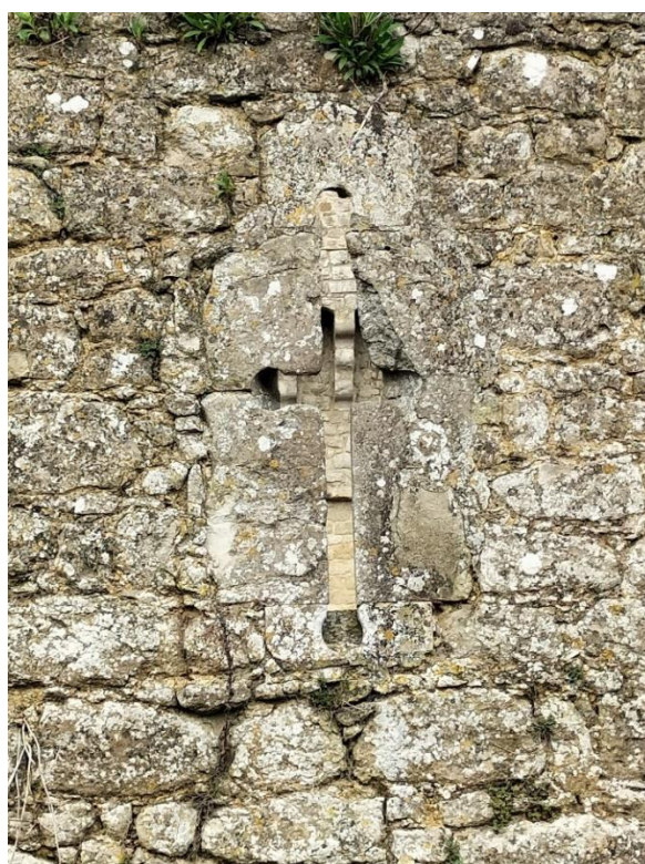
Fig. 107: Fully-oilleted cross-loop in the barbican at Leeds Castle
