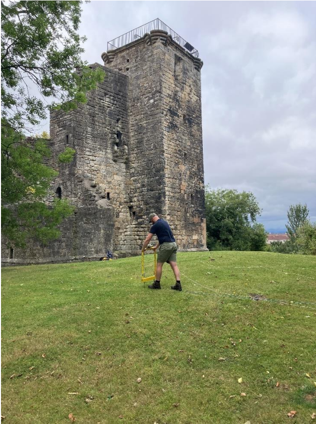
Image 5 - View of areas CK04 and CK08 looking north ( DP626677 )
